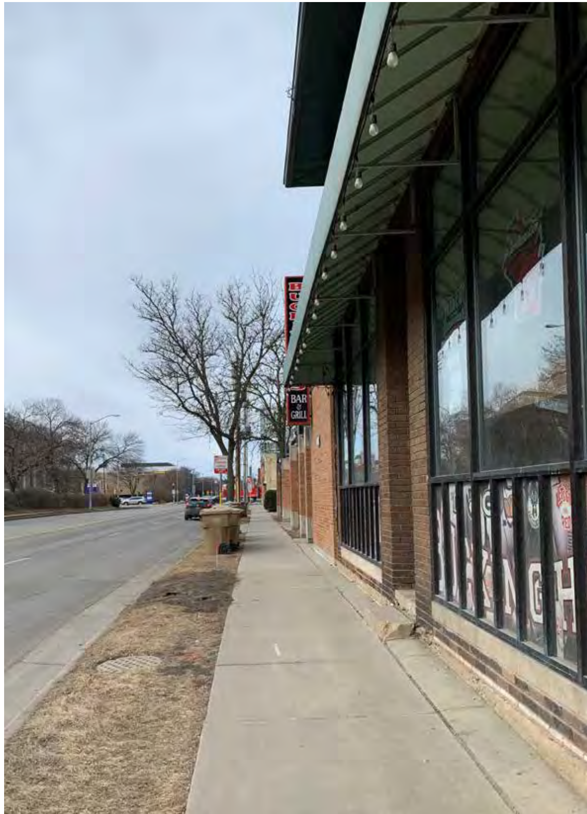
EXISTING SIDEWALK CONDITION ALONG REGENT (APPR. 7' FROM CURB TO BLDG.)
