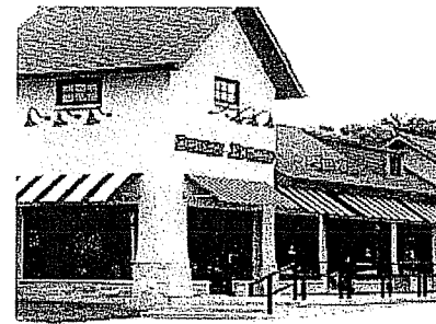
Small retail and office development on Madison's west side is adjacent to senior and condominium housing.
