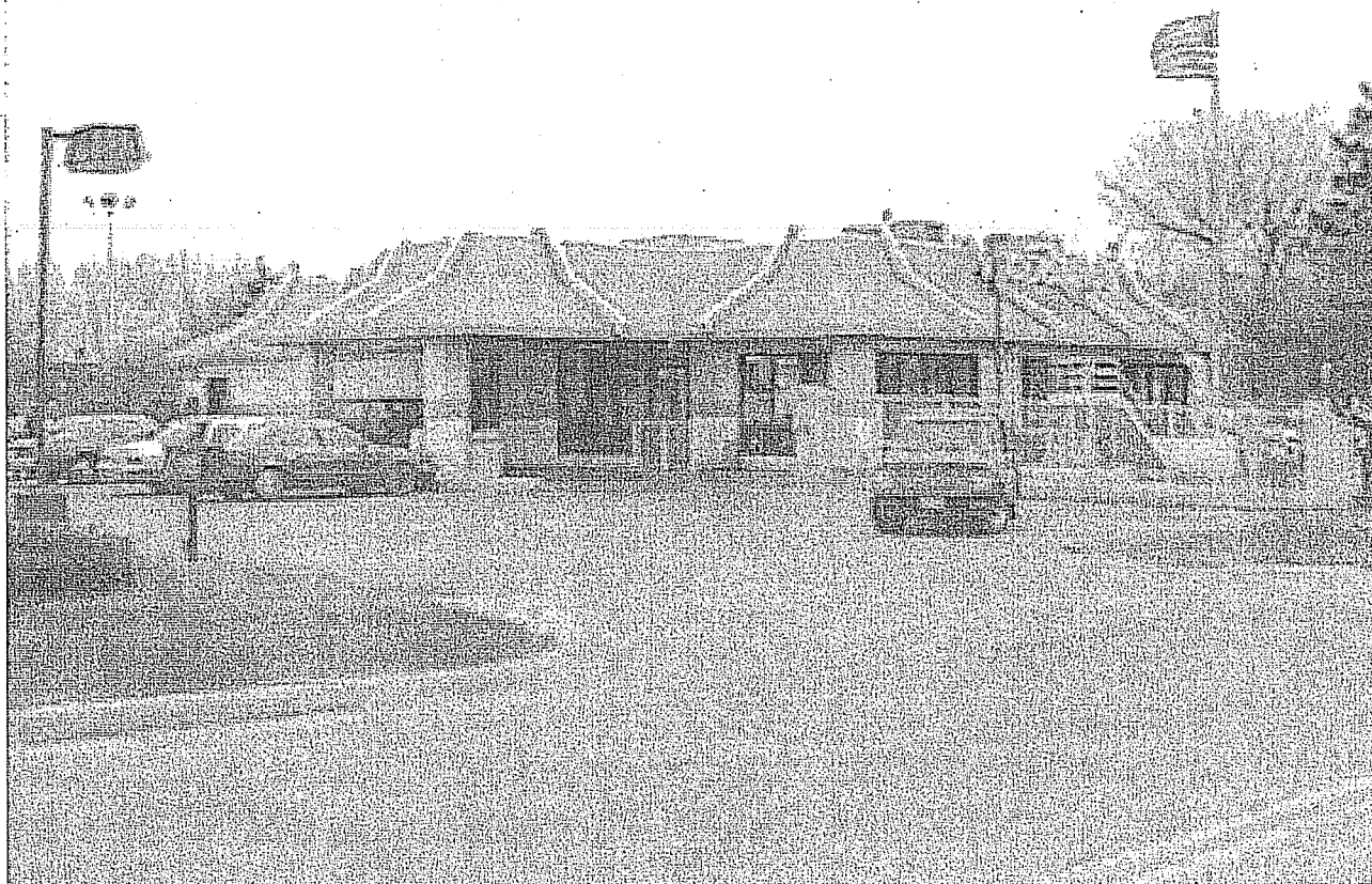
3051 E. Washington Avenue McDonalds proposed for demolition for new McDonalds
