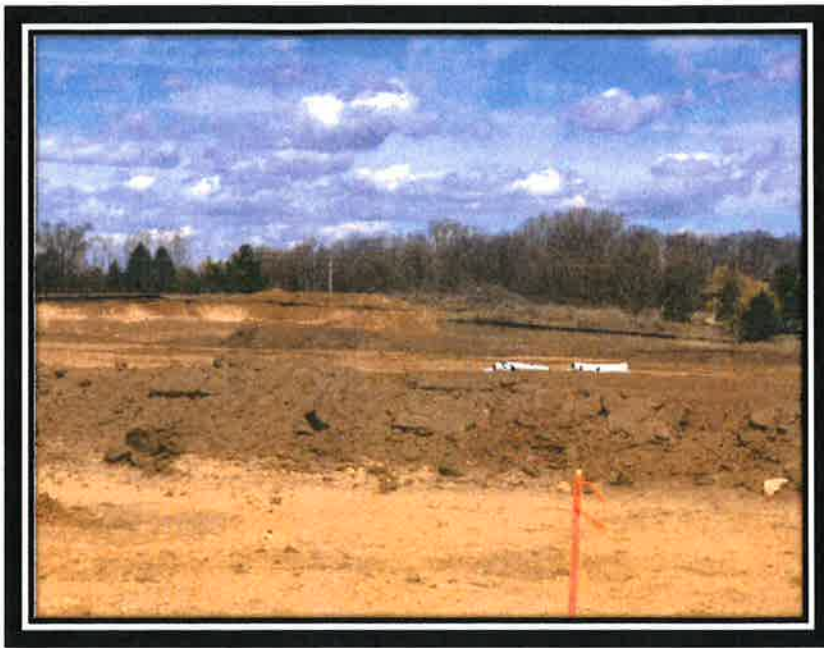
Site View Looking North from White Fox Lane at Dragon Willow Lane
