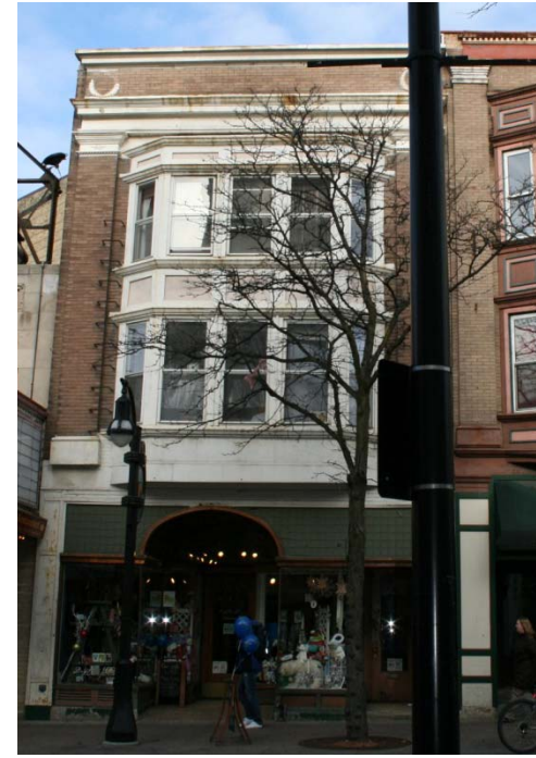
Schumacher Building (214 State Street)
