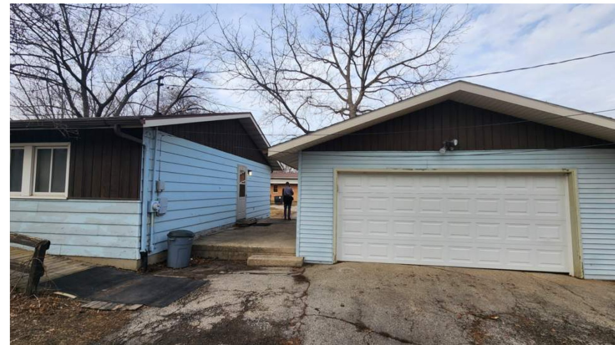
1982 food pantry garage, South facade
