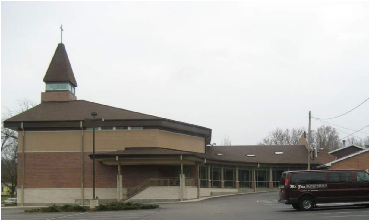
2004 construction, North entrance
