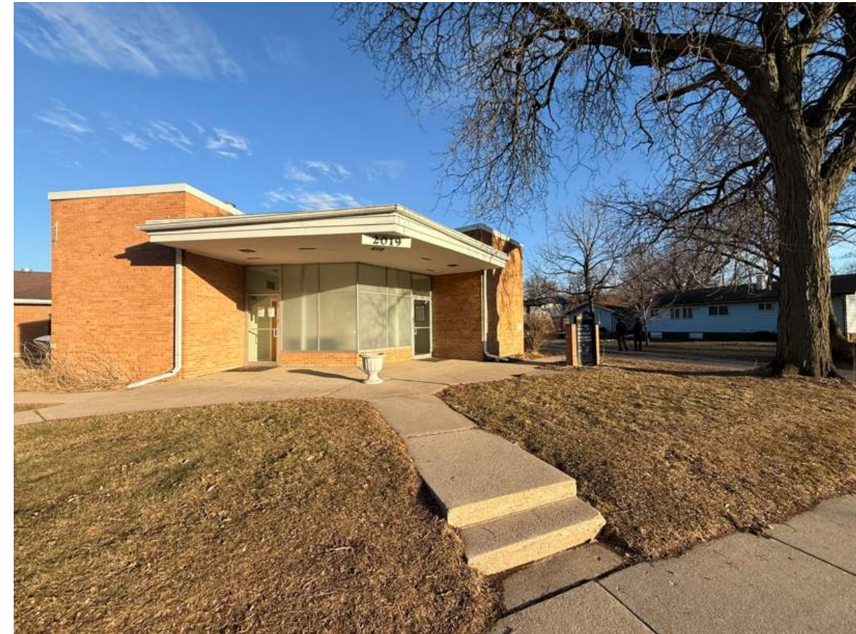
1961 construction, Main (West) entrance
