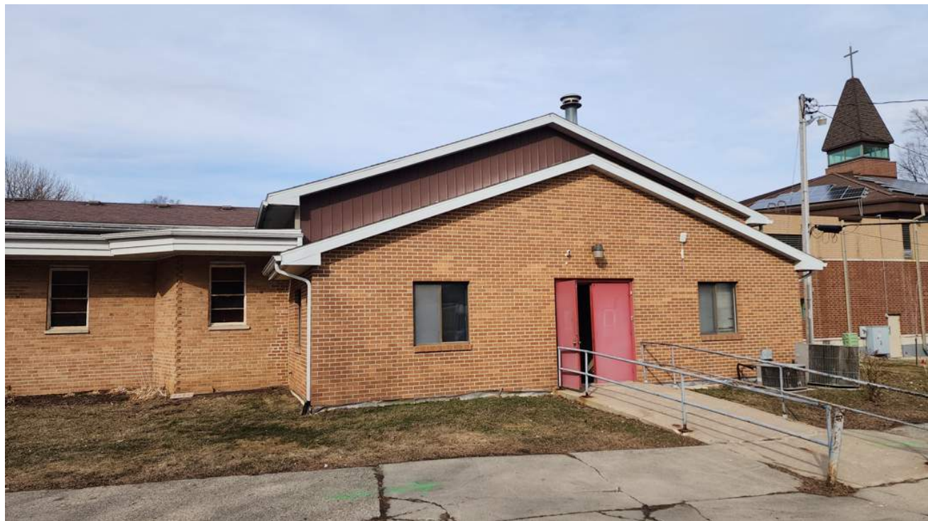
1961 construction, South entrance
