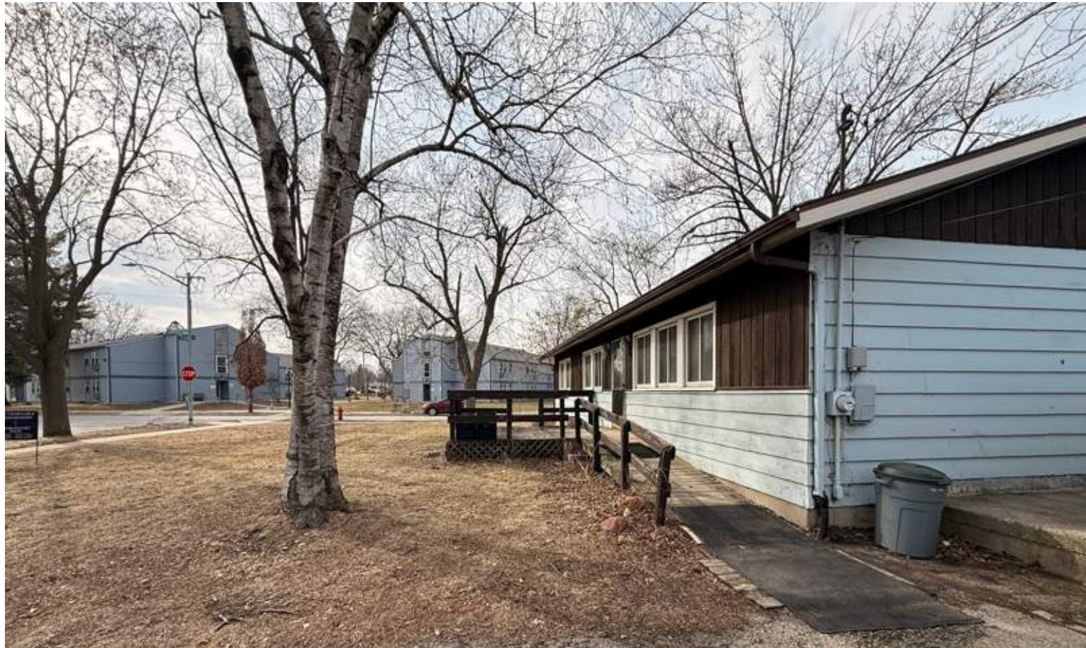
1982 Food Pantry, South facade and entrance
