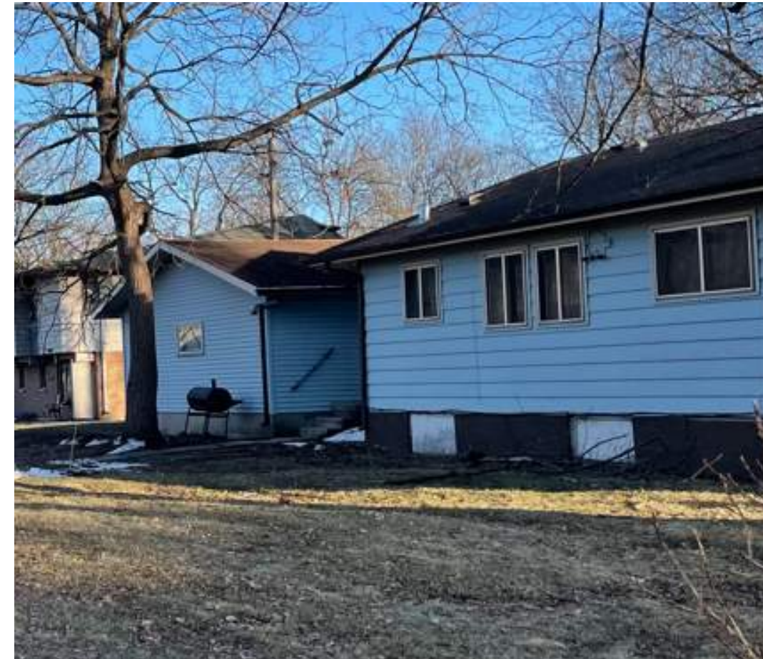
1982 Food Pantry and garage, North facade
