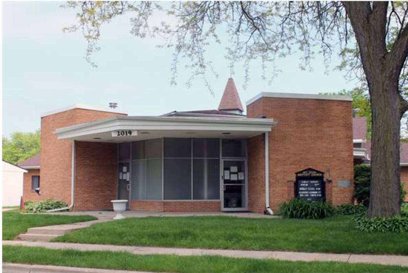
1961 construction, Main (West) entrance
