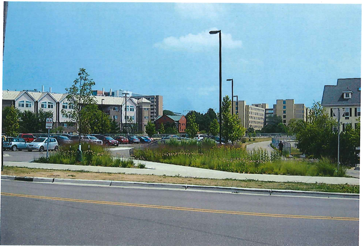
Completed Parking Lot, Summer 2013 (View NE)
