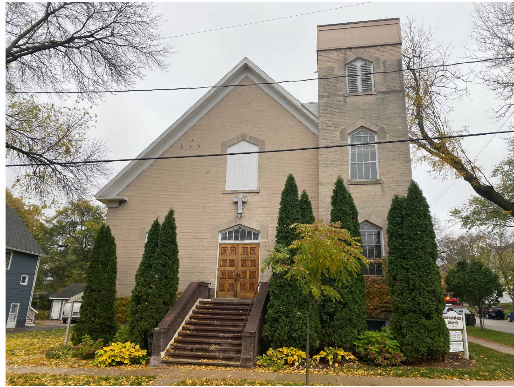
PHOTO 4: LOT 1 EXISTING CHURCH: 1103 JENIFER ST: STREET ENTRY- JENIFER ST.
