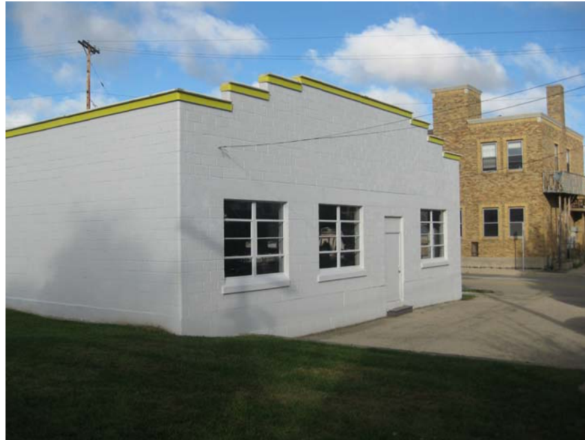
VIEW FROM 967 SOUTH PARK STREET LOOKING NORTH
