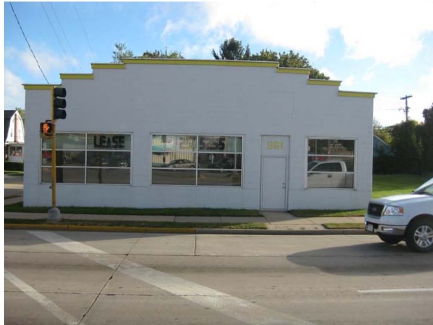
VIEW FROM PARK STREET LOOKING EAST
