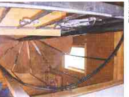
Stair Down to 2nd Floor
