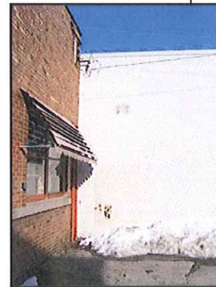
EXISTING AWNINGS AND ADJACENT BUILDING
