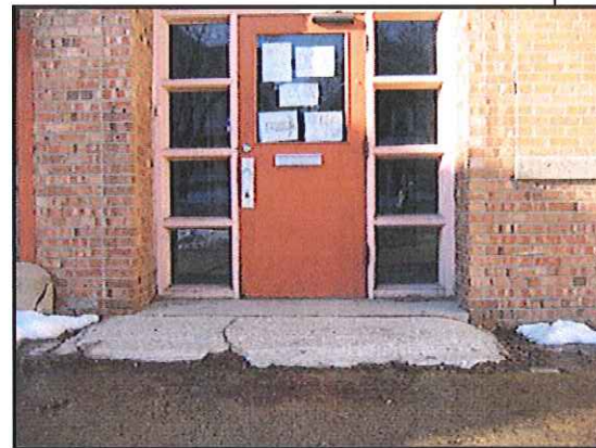
EXISTING ENTRY DOOR AND SLOPED STOOP
