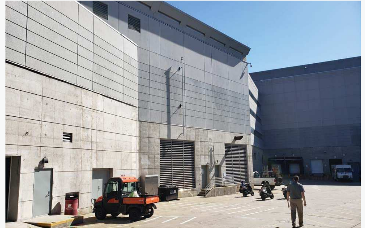
View into Kohl Center loading area
