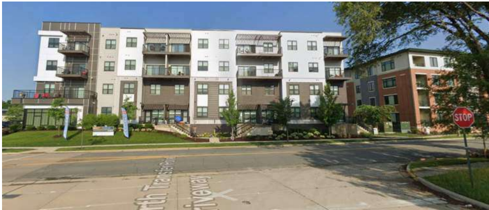
Building Across: 1201 Huxley St
