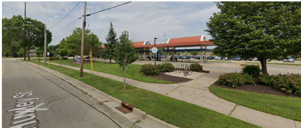
VIEW FROM SOUTH TO NORTH
