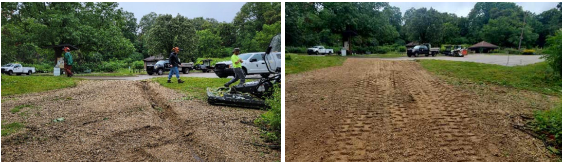
Gully and erosion repair at Owen.
