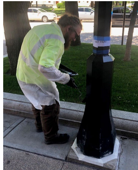
Mall employee painting light post
