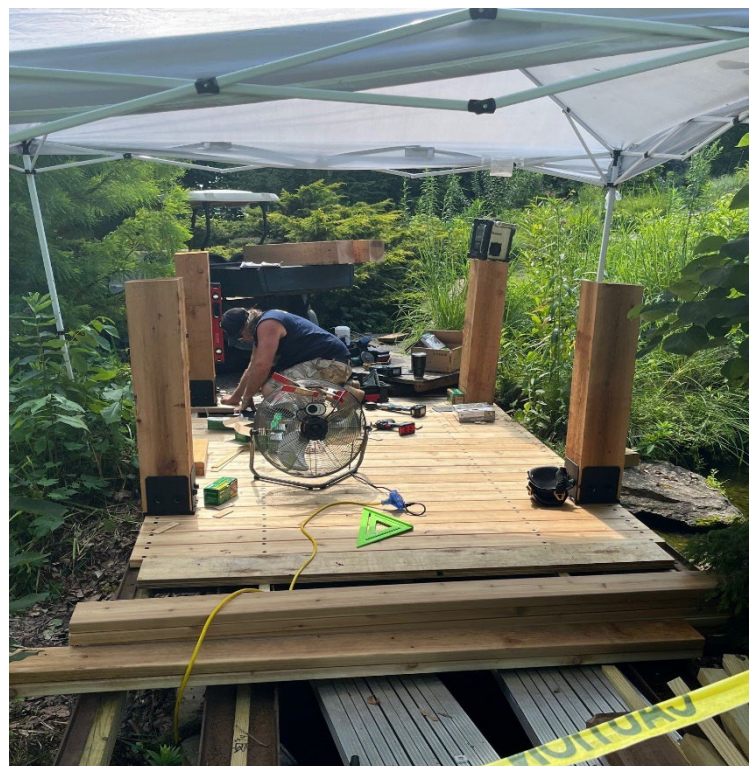
Olbrich bridge rebuild
