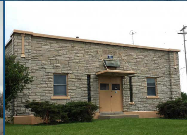
Unit Well #12 Generator Project Status: Completed | Investment: $40 thousand
