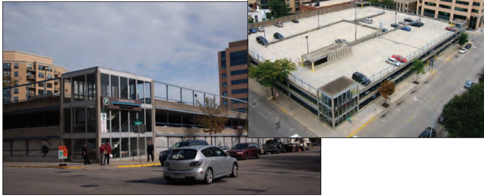
Government East Parking Garage, 2012
