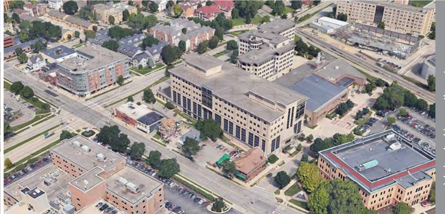
aerial view looking northwest
