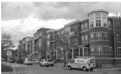
Figure D6: Building Alignment
