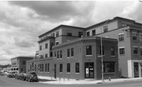
Figure D4: Variation in Roof Lines
