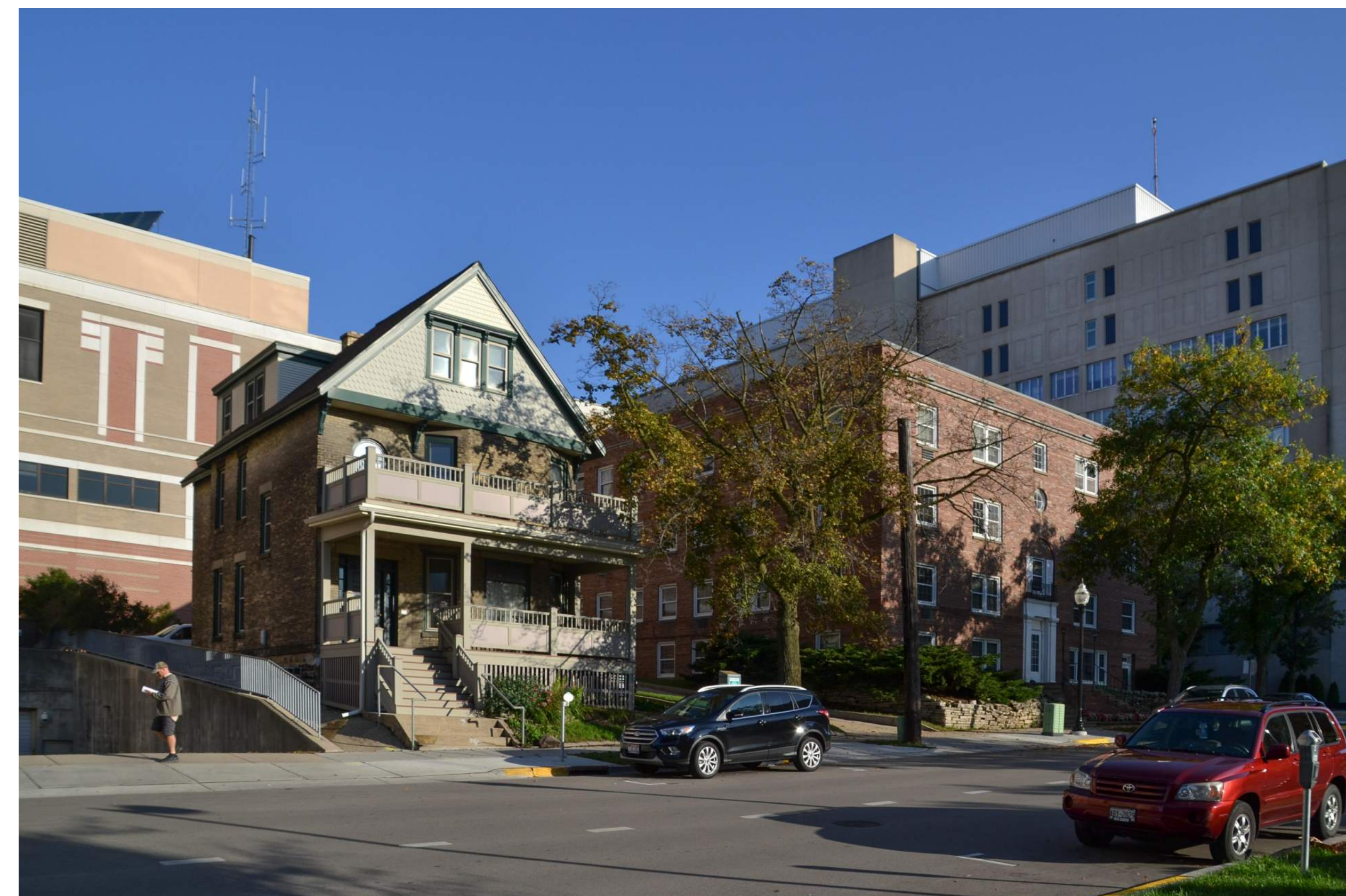
View of 112 West Wilson Street
