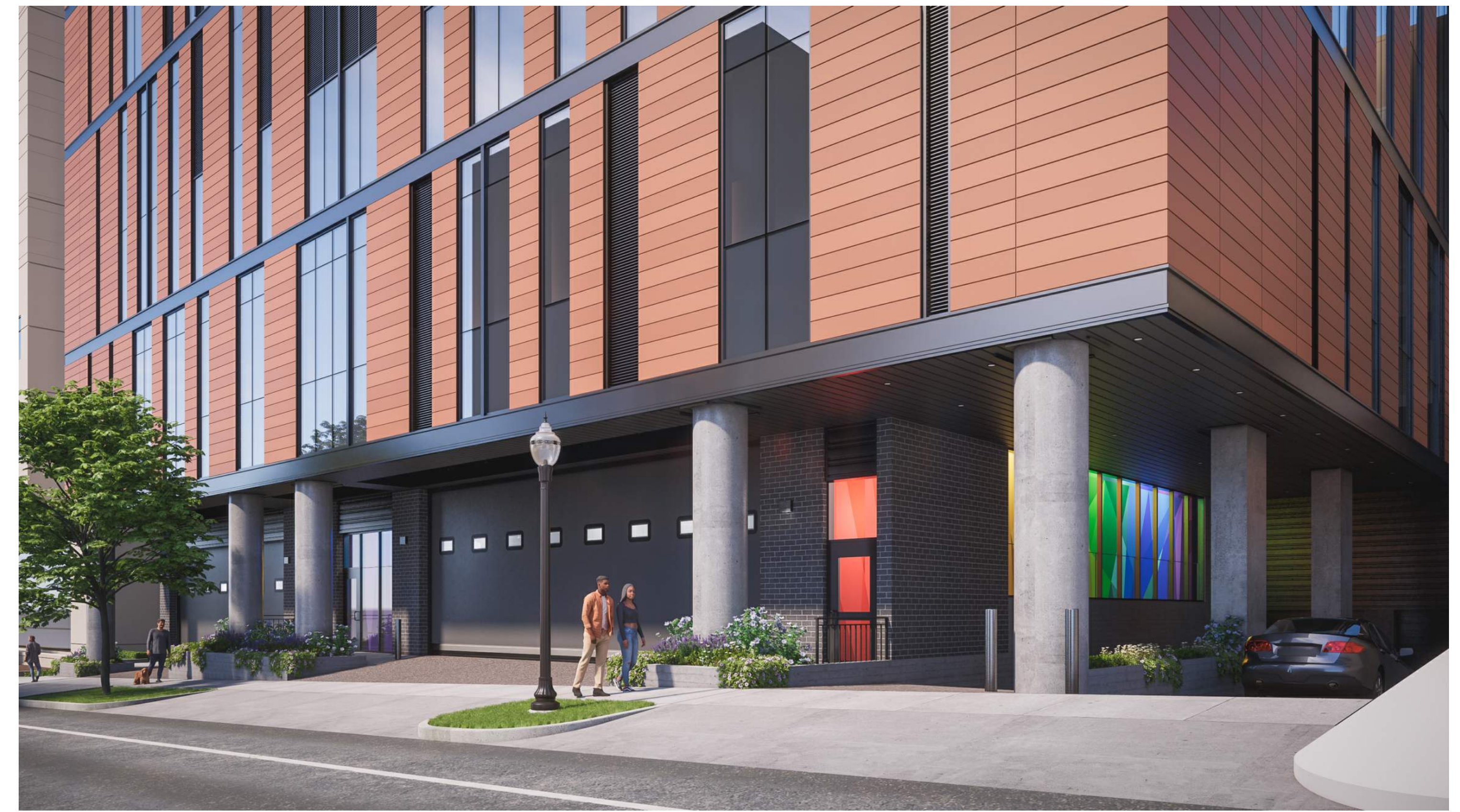
STREET LEVEL EAST
