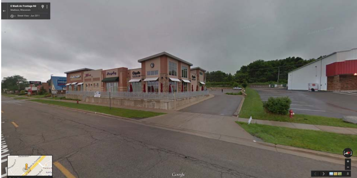
The existing building to the west. Predominately an EIFS/Masonry multi-tenant building.
