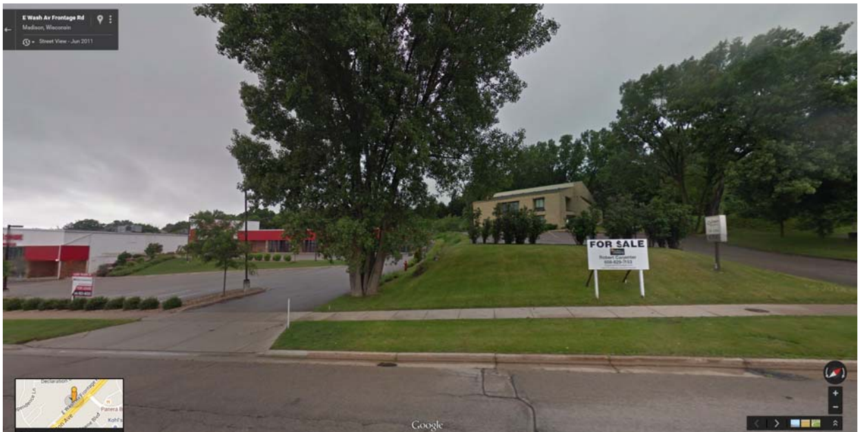
The existing office building to the east.
