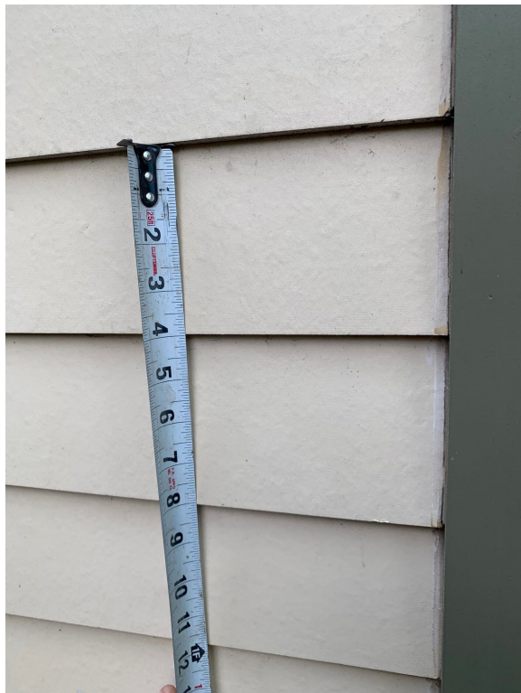
Picture showing the overlap of the siding.
