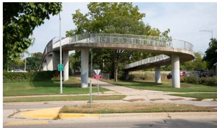
A pedestrian/bike bridge crosses Stoughton Road 900 feet south of Milwaukee Street
