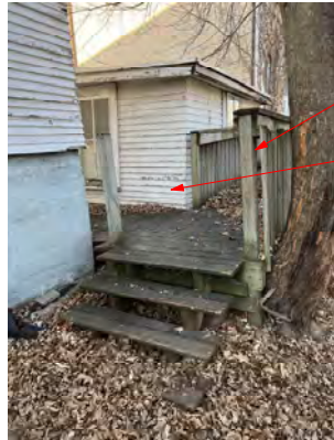
PHOTO 6: VIEW OF ACCESS RAMP PORTION FROM BEHIND LOT 2
