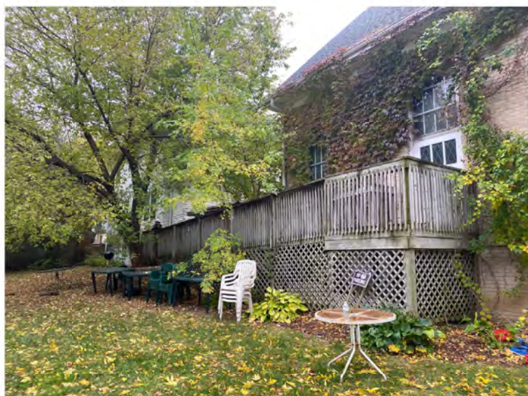
PHOTO 6: LOT 3 (FOREGROUND) LOT 1 (BACKGROUND) EXISTING CHURCH SIDE- EXISTING ACCESS RAMP
