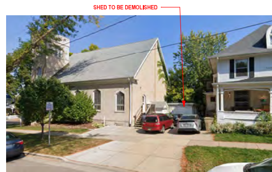
PHOTO 1: DRIVEWAY ACCESS TO 511 INGERSOLL
