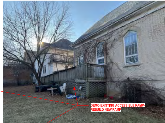
PHOTO 7: EXISTING ACCESSIBLE RAMP TO CHURCH
