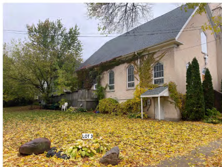
PHOTO 5: LOT 3 (FOREGROUND) LOT 1 (BACKGROUND) EXISTING CHURCH SIDE
