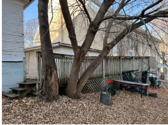
PHOTO 8: EXISTING ACCESSIBLE RAMP TO CHURCH
