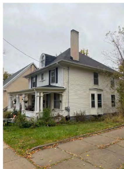
PHOTO 1: LOT 2 EXISTING HOUSE: 511 S. INGERSOLL ST
