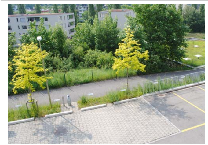
Permeable parking strip drains to grassy swale to protect stream quality, Futuro Office Park in Liestal Switzerland Photo Laura Tam
