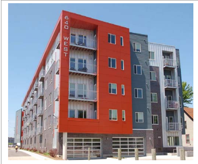
Five-story apartments at 640 W. Wilson St. in Madison, WI
