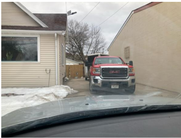
January 30 th , 2024, 4pm – Construction truck and trailer obscuring entire driveway.
