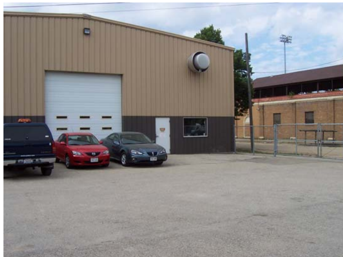
Northwest – Collision Repair Center
