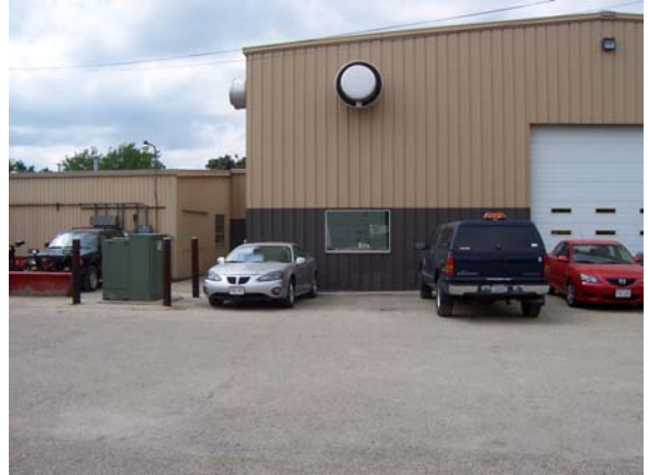
Northwest – Collision Repair Center
