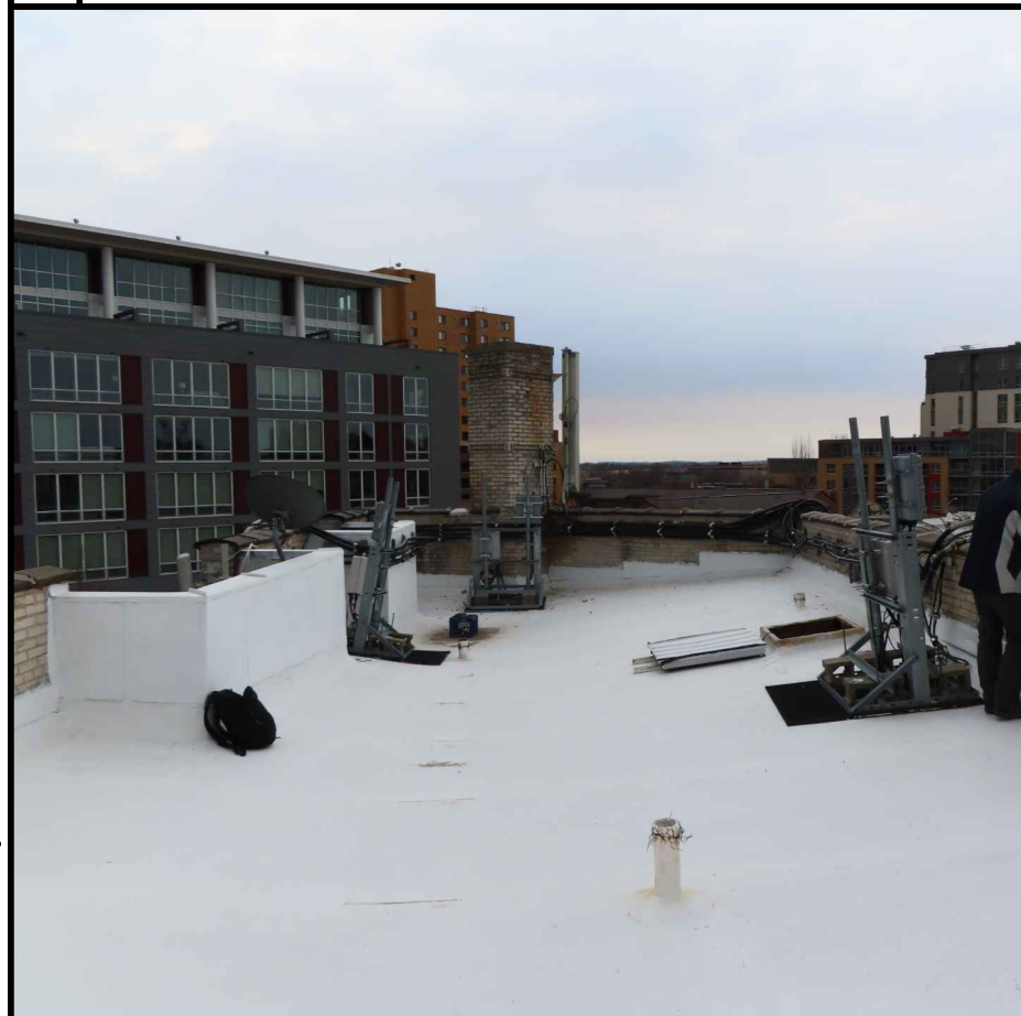
D EXISTING ROOFTOP OVERVIEW
