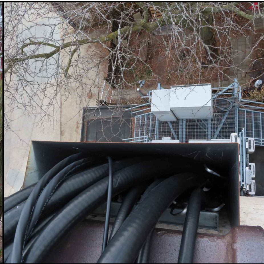
B EXISTING CABLE ROUTING UP BUILDING EXTERIOR
