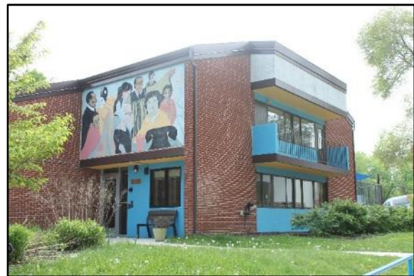
South Madison Day Care Center 2012 Fisher Street
