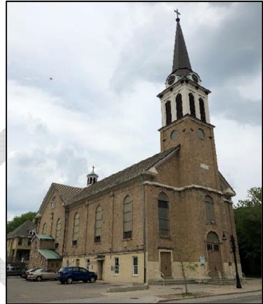
Holy Redeemer Parish Catholic Church 128-132 W. Johnson Street
