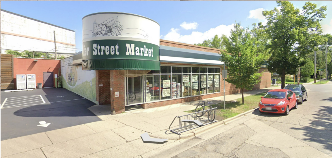
EXISTING STREET VIEW
