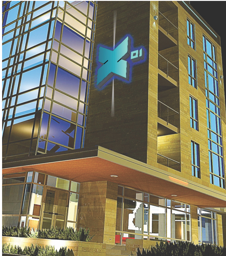
X01 building with cabinet letters on building showing Led blue halo
