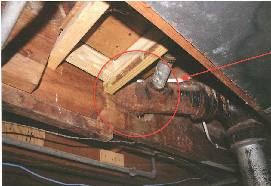
Cutting of joists
