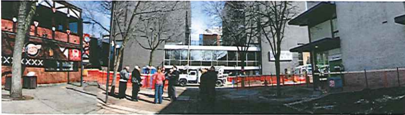
Early spring 2008 site conditions at Frances Plaza, looking south and north
