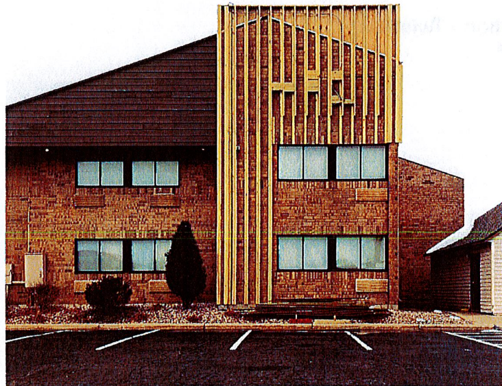
Reinstalled existing Building Letters facing new façade on W. Beltline Hwy. (South) Elevation
