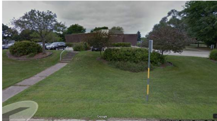
View to West of Existing Building from Huxley St.
