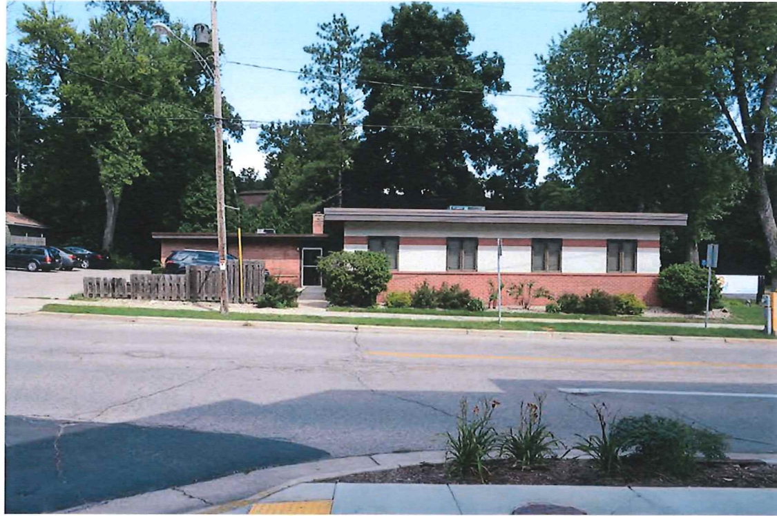
Existing Building along Glenway Street
