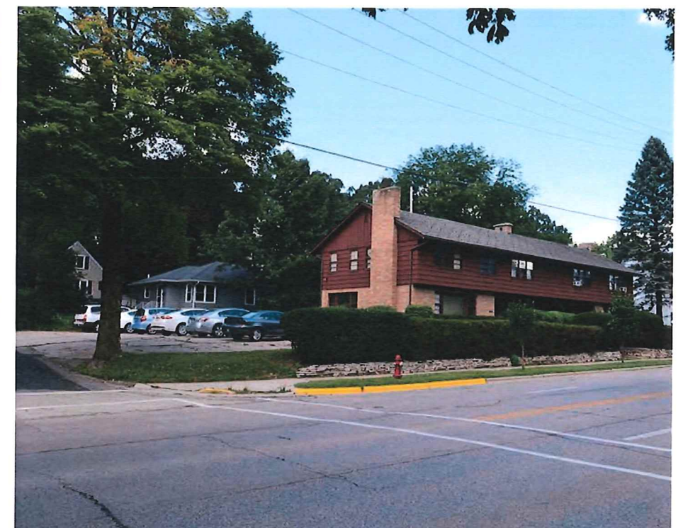
Apartments along Monroe Street east of Arbor House
