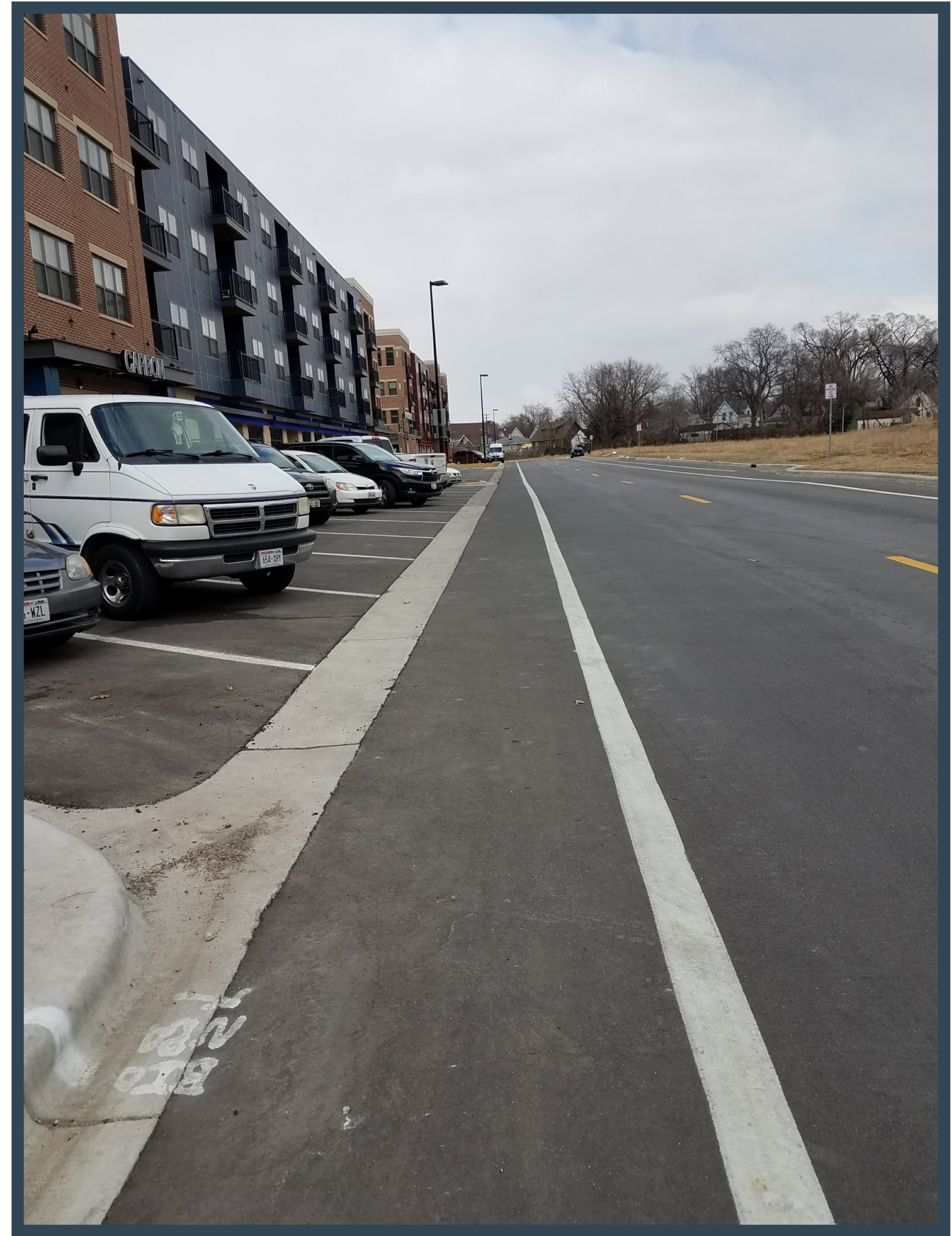
BICYCLE LANE ON NORTH SIDE OF WINNEBAGO STREET
