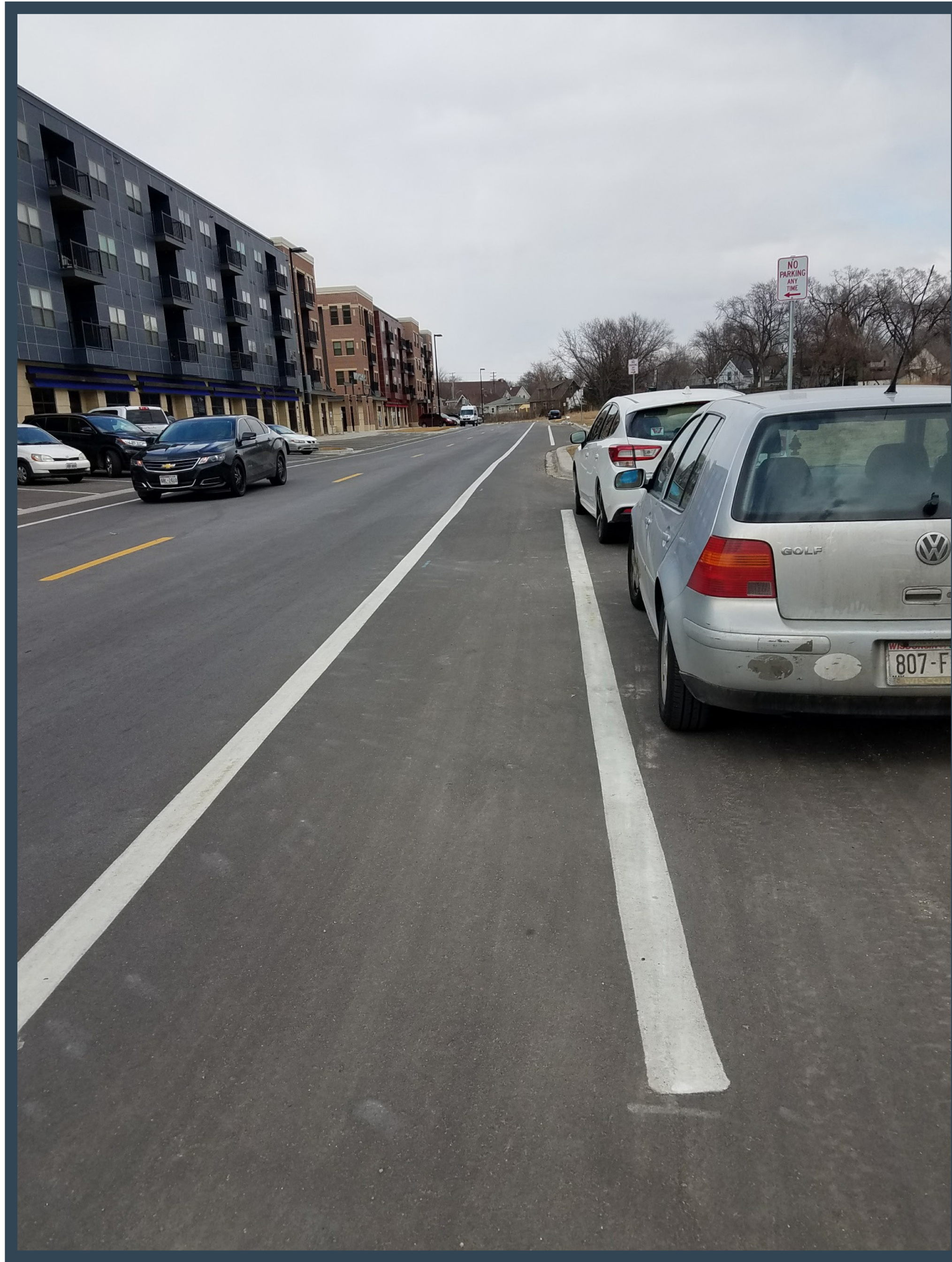
BICYCLE LANE ON SOUTH SIDE OF WINNEBAGO STREET
