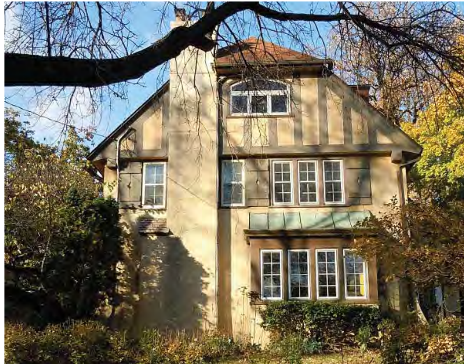
L: 2110 Chadbourne Ave Roof: Gambrel Hip Facing Front Facade: Stucco, Vertical Exposed Timbers
