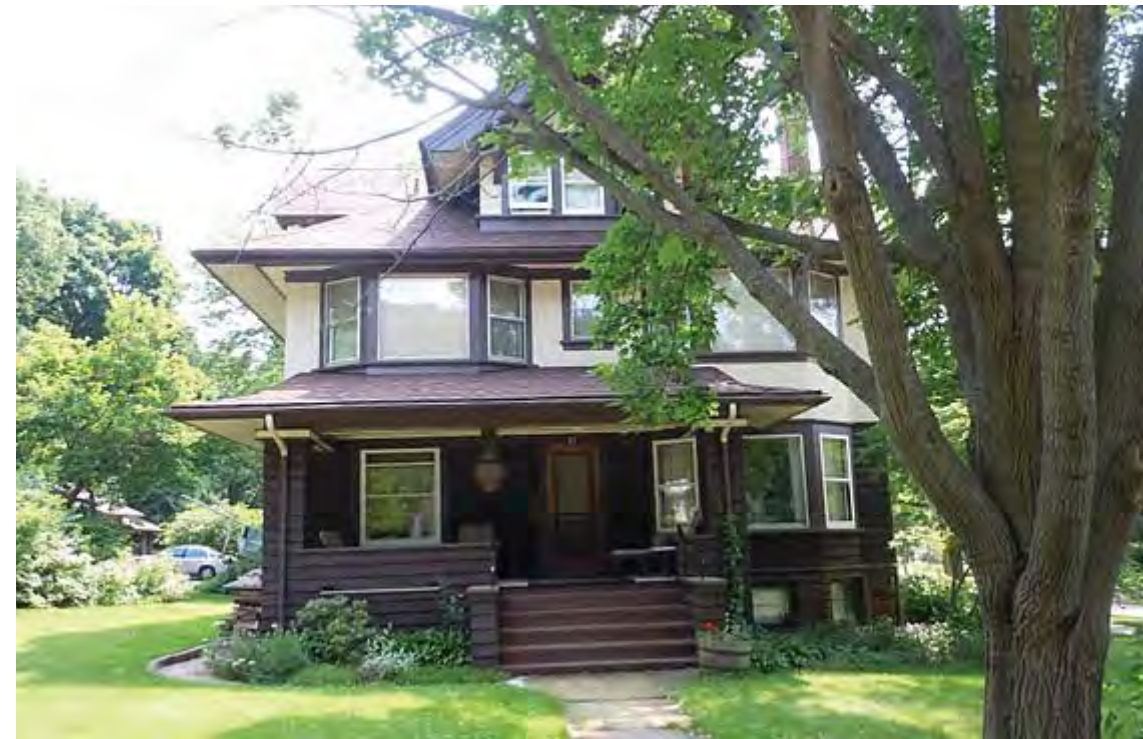
B: 21 North Prospect Ave (adjacent to proposed structure) Roof: Hip, Deep Overhang Facade: Stucco, Horizontal Wood Siding
