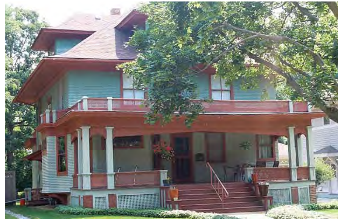
M: 15 North Prospect Ave Roof: Hip, Deep Overhang + Flat Roof Porch Facade: Horizontal Wood Siding
