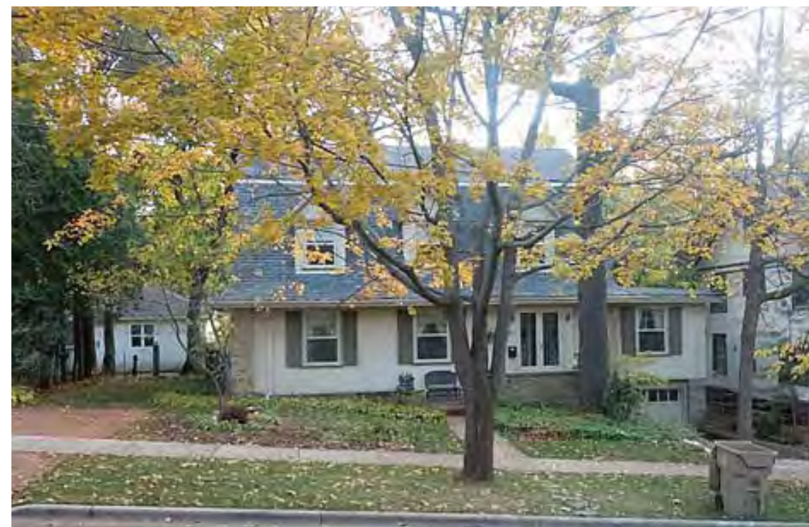
F: 2111 Van Hise Ave Roof: High Gambrel, Facing Side + Garage Flat Roof Facade: Stucco, Stone
