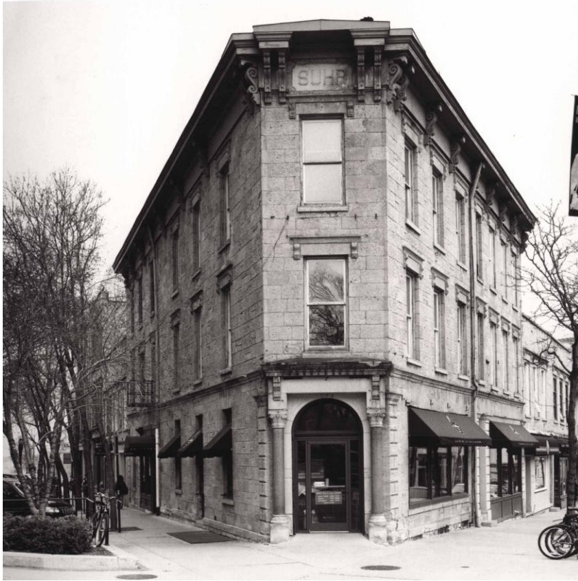
The Suhr Building 2001 (Zane Williams)
