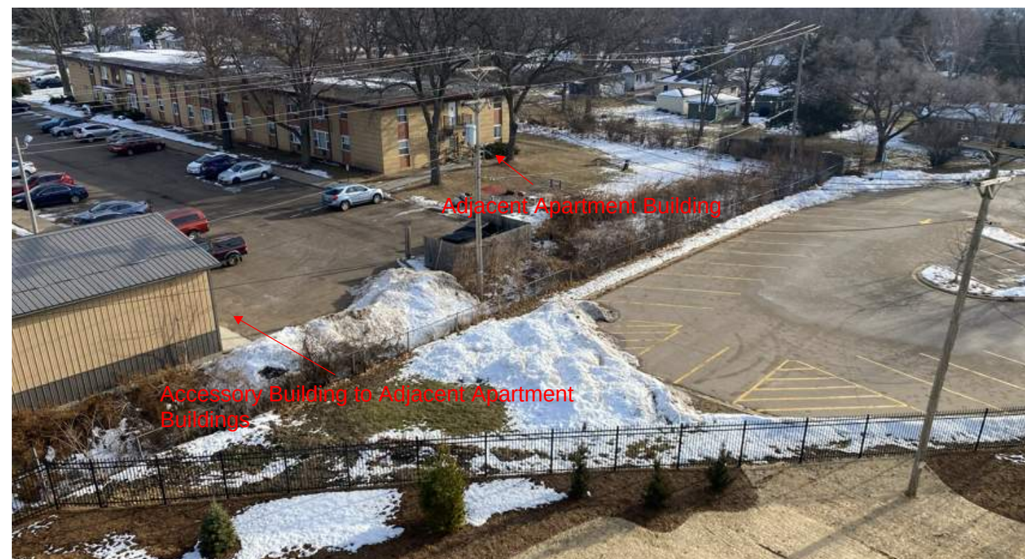
Segment C 3 Aerial
