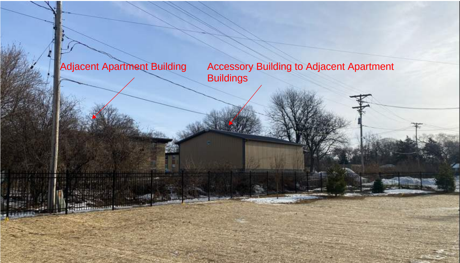
Segment B and Part of C 2
