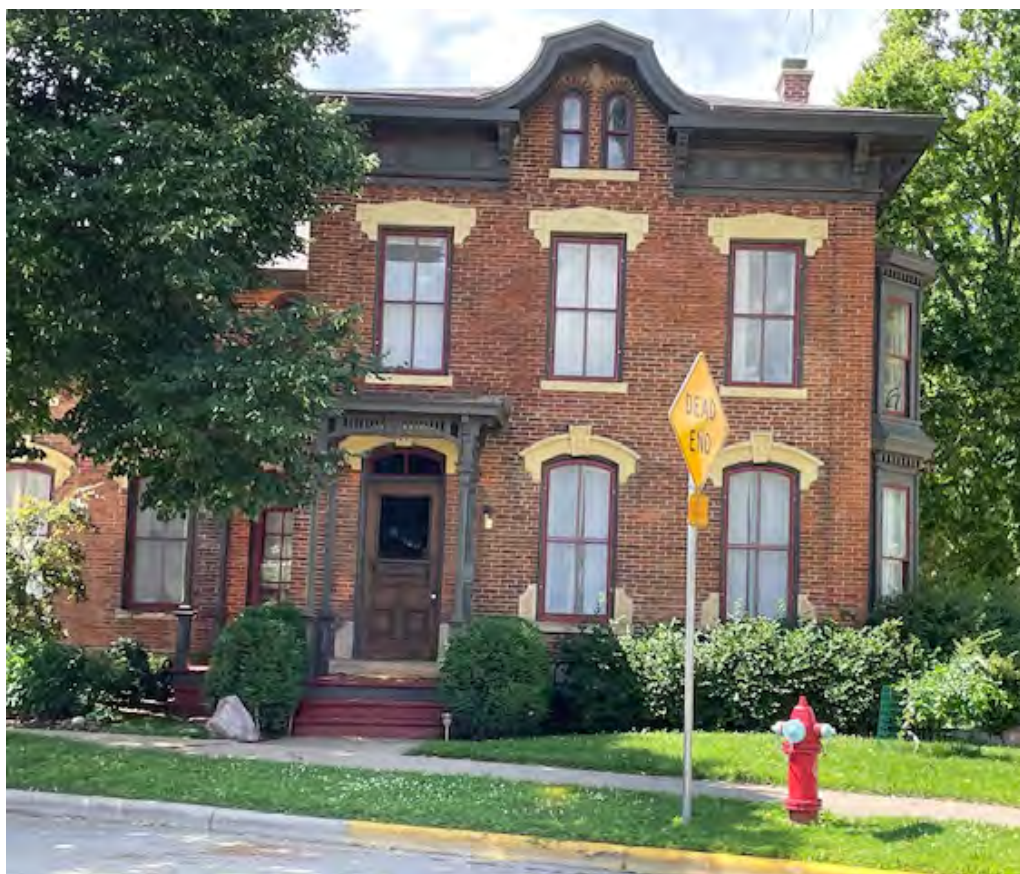
Ott House (north-east kitty-corner of residence)
