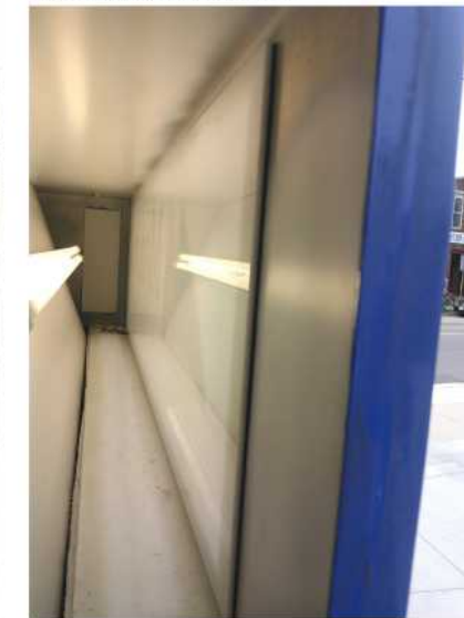
INSIDE VIEW OF EXISTING FACE
