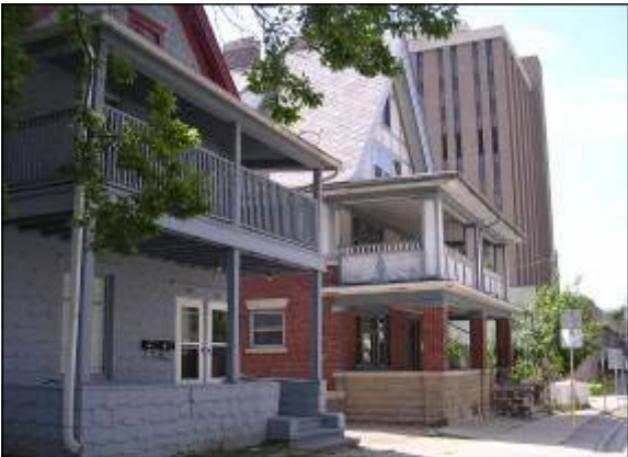
■ Student housing adjacent to University facilities north of the planning area.
