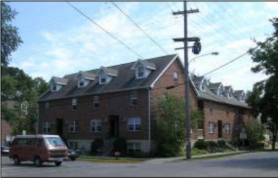
■ Typical student housing development north of Regent Street.
