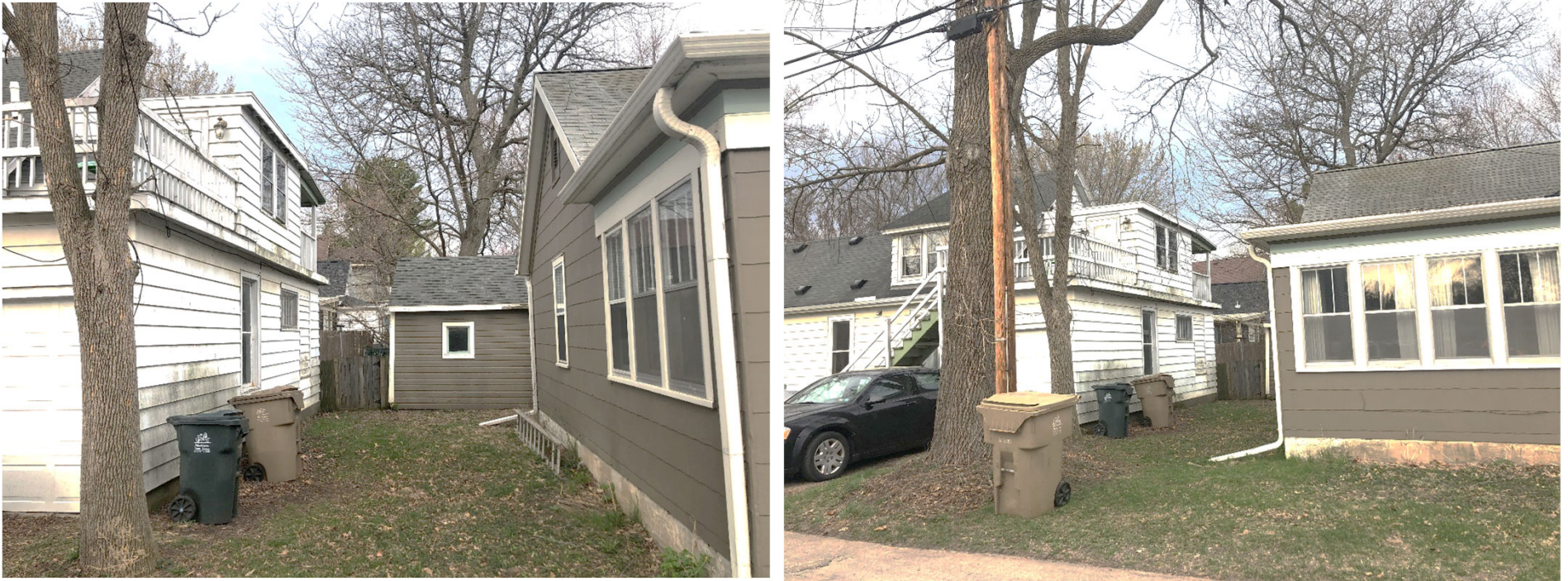
VIEWS OF REAR YARD AREA AND AREA BETWEEN BUILDINGS, FROM ALLEY
