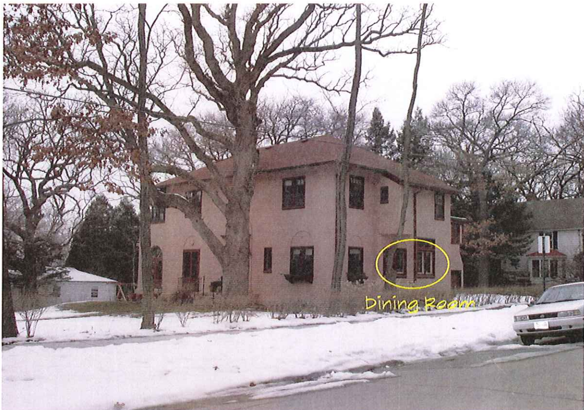
southeast & East facing dining room windows
