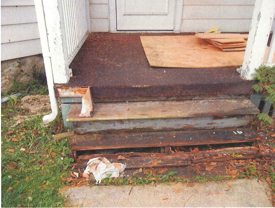
Surrounding properties: On Rogers Street
