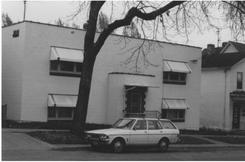
134 S. Franklin St, built 1940
