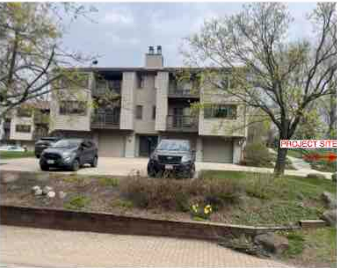
EXISTING 3 LEVEL - STACKED 4 CONDOS - SOUTH VIEW TOWARD STREET GRADE LEVEL 1 CAR GARAGE
