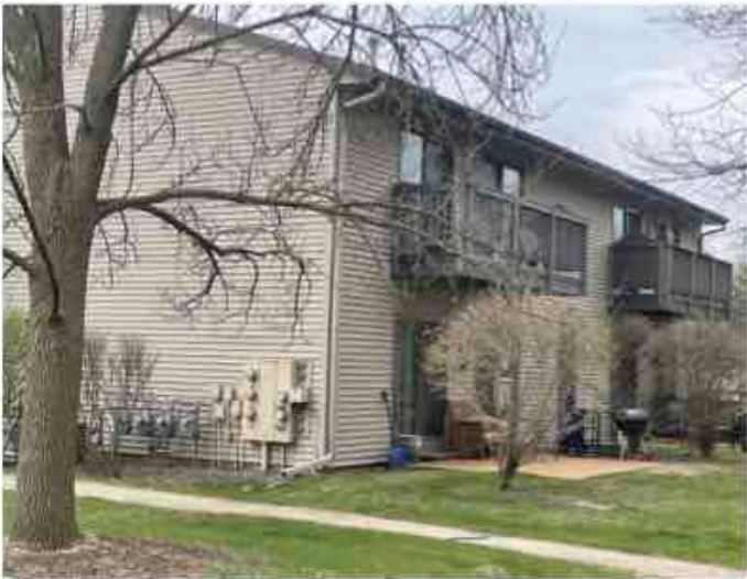
EXISTING 3 LEVEL - STACKED 4 CONDOS - NORTH VIEW TOWARD POOL
