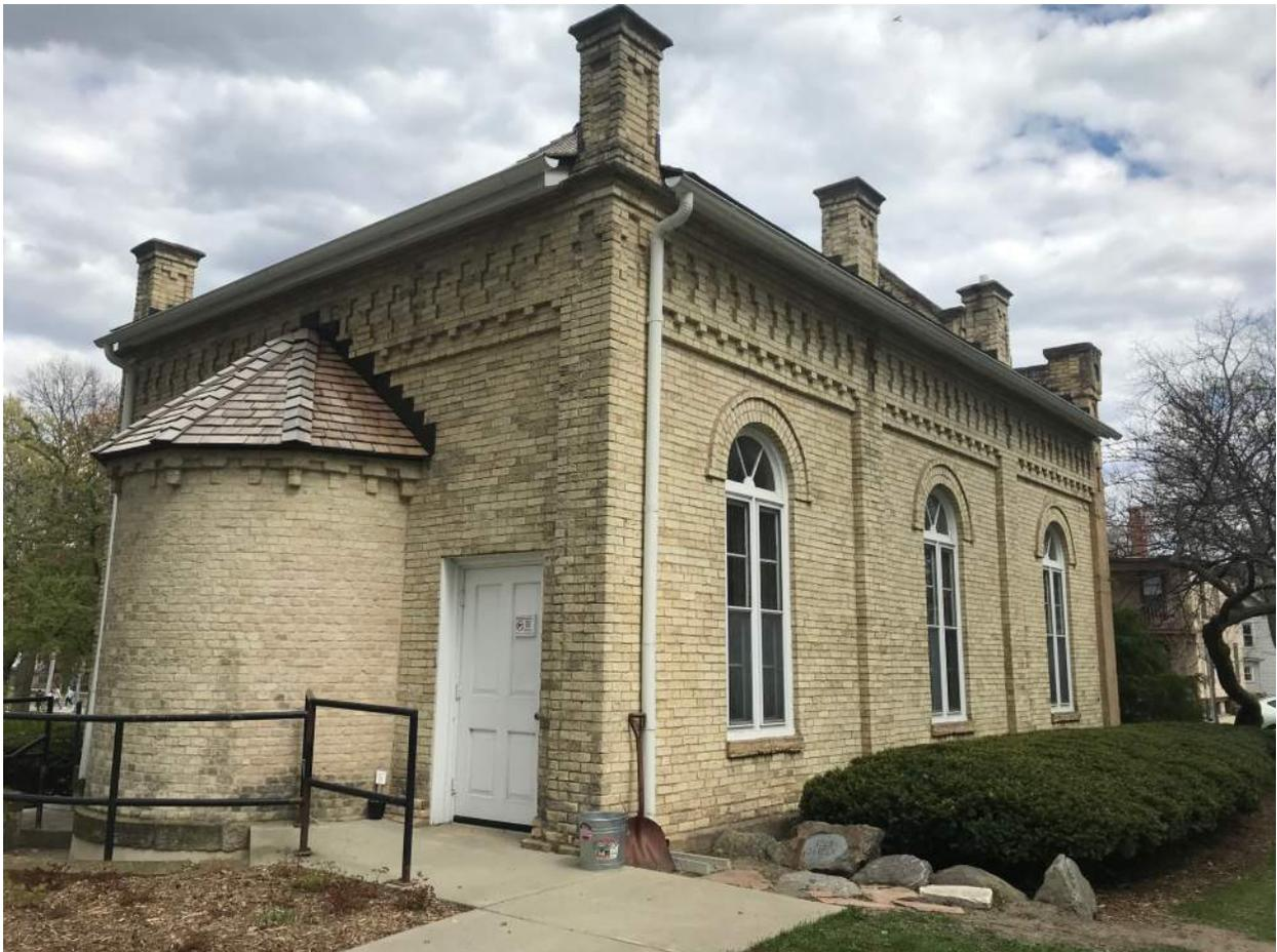
Gates of Heaven northwest corner showing condition of brick and windows. Brick of apse was recently repointed.
