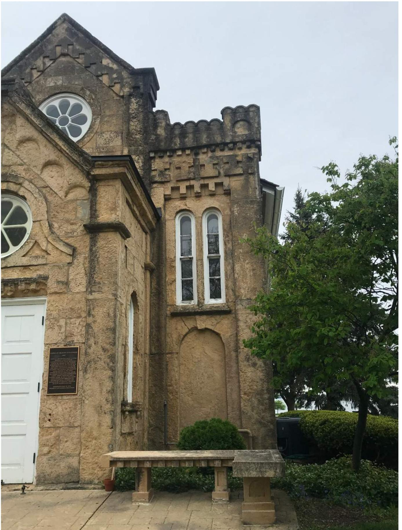
Gates of Heaven southeast portion of front facade showing condition of stone and discoloration. Also note condition of windows and lack of protective storm windows on some windows.
