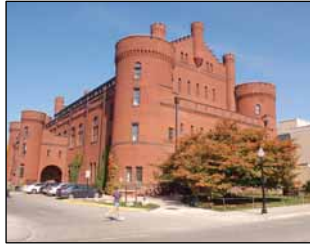
UW Armory and Gymnasium
