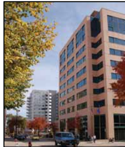
State Department of Administration Building
