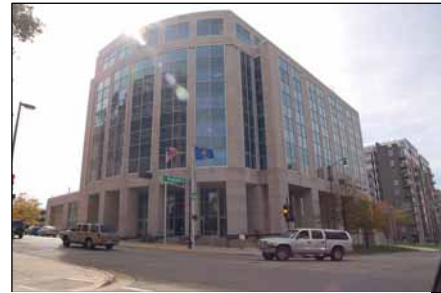
Tommy Thompson State Office Building
