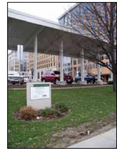
A solar canopy
