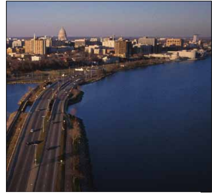
John Nolen Drive corridor causeway
