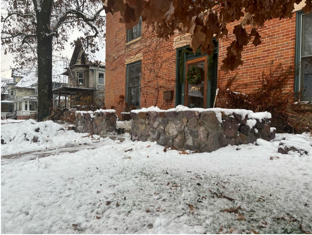
Existing Patio Wall
