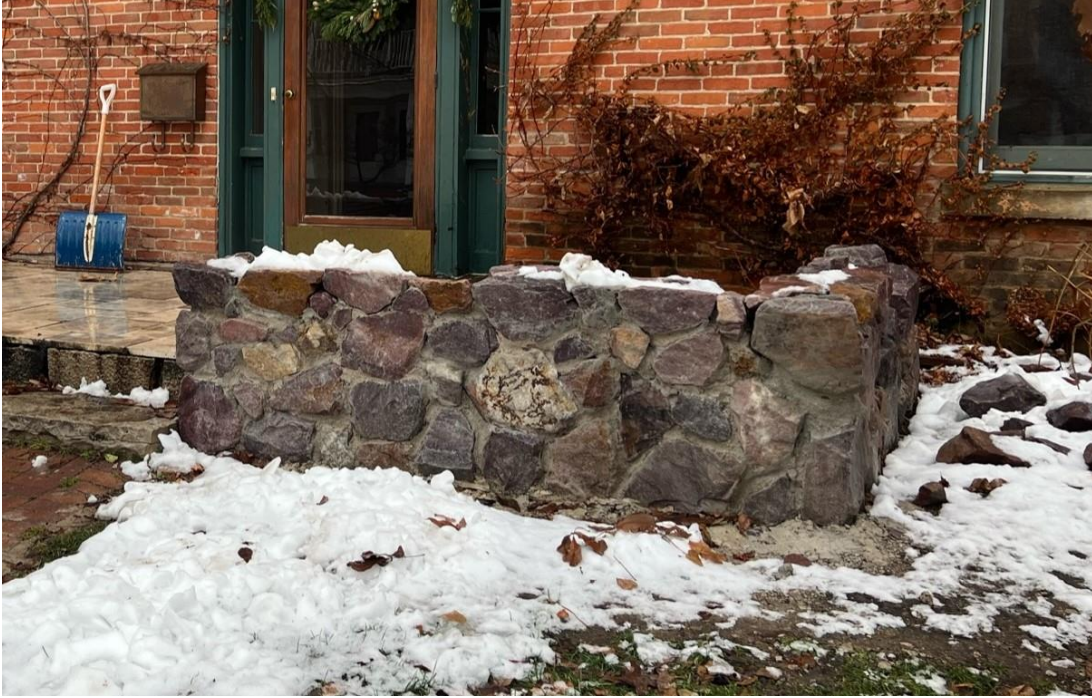
Existing Patio Wall
